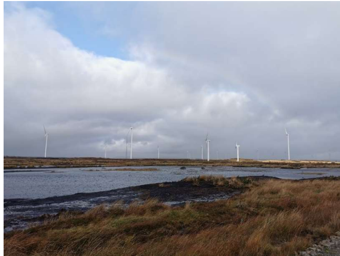
Figure 2.3: Existing Bellacorick Wind Turbines
